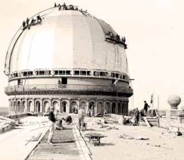
▲ TOPPING IT OFF The great dome of Yerkes Observatory was tinned and cemented in the autumn of 1896.
